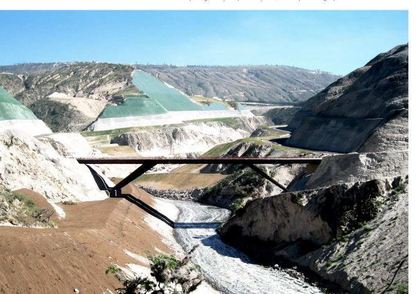
the deck has been launched from the top and finally the last spans have been installed by using crawler cranes.
